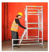
4) CLIP UPPER BRACE OF LADDER ABOVE RINGS ON VERTICALS WITH ASSEM-BLED HOOKS AT TOP
